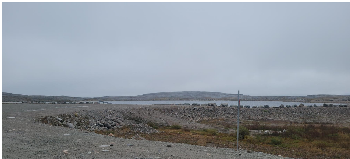
Figure 4: View of the non-aerated lagoon
