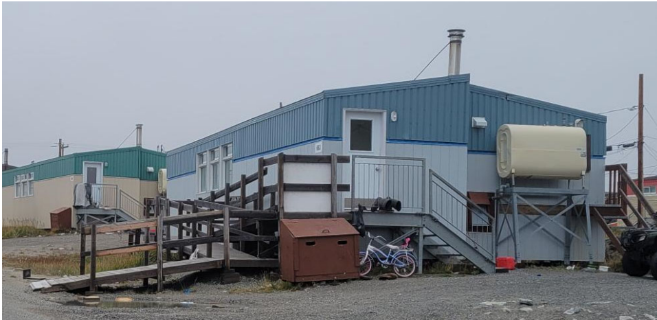
Figure 5: Example of a house, a container for residual materials, and a heating oil tank
